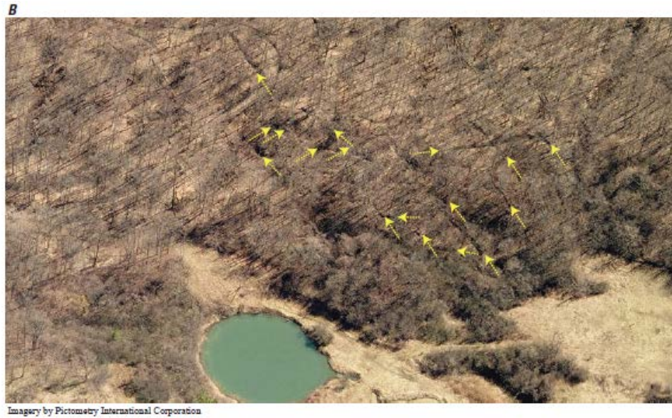
Figure 4. Hillside fissures are visible in this leaf-off aerial photograph (from Hackett et al., 2009).
